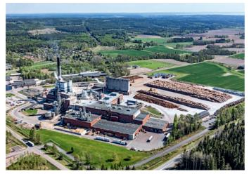
In **Bäckhammar**, our two paper machines produce more than 159,000 tonnes of unbleached Kraft paper every year. And our pulp mill at Bäckhammar produces more than 230,000 tonnes of unbleached pulp a year.
